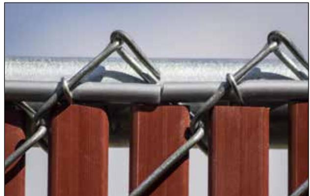
**Do not overlap the noodle, make sure the noodle ends are touching and then hog ring tightly. The hog rings must be very, very tight to prevent the noodle from moving in the wire.**
