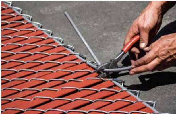
Cut the excess noodle halfway between the two selvages where the two rolls or sections come together, so both ends of the noodle touch. Using the hog ring pliers, hog ring both ends of the noodle to the wire very tightly, making sure both ends are still touching. Keeping the noodle secure from moving in the wire.
