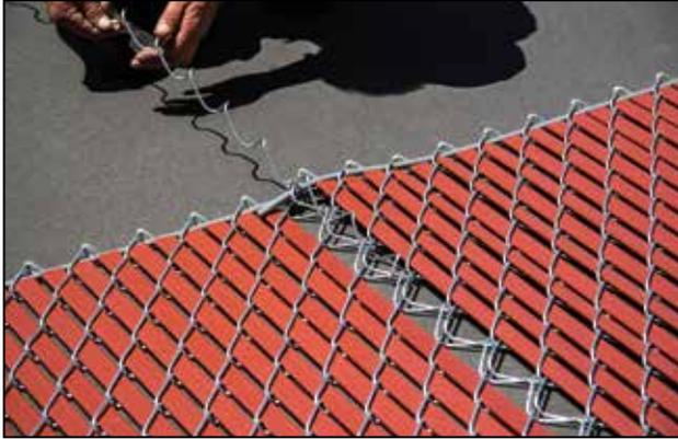
Insert the needle and connect the rolls same as regular chain link fence. Stand the fence up to the posts and top rail, loosely attach to the top rail, attach tension bar and stretch wire into place. **Do not cut the noodle until you have stretched the wire.**
