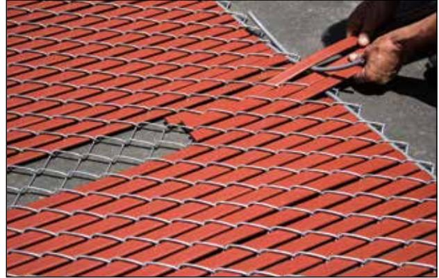
Install the three (3) slats that come with each roll in the space created as a result of hooking the two rolls or sections together with the wire needle provided.
