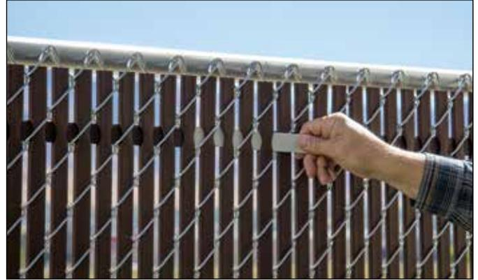
How to install the three (3) extra slats in place between spliced sections: Cut the 8" Flat Noodle tail off the end of the roll. Insert one slat at a time while feeding the Flat Noodle tail into place until all three slats are inserted. Make sure the Flat Noodle from the tail overlaps the other Flat Noodle where the extra slats were installed.
