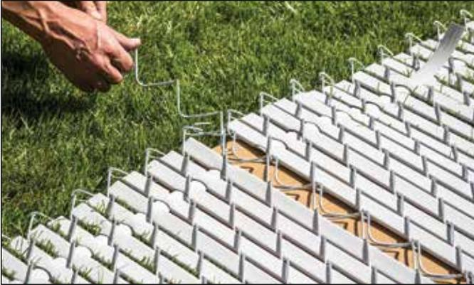
Insert the needle and connect the rolls of Flat Noodle Link the same as regular chain link fence. Stand the fence up to the posts and top rail, loosely attach to the top rail with ties. Attach tension bar and stretch wire into place. **Do not cut the Flat Noodle until you have stretched the wire.**
